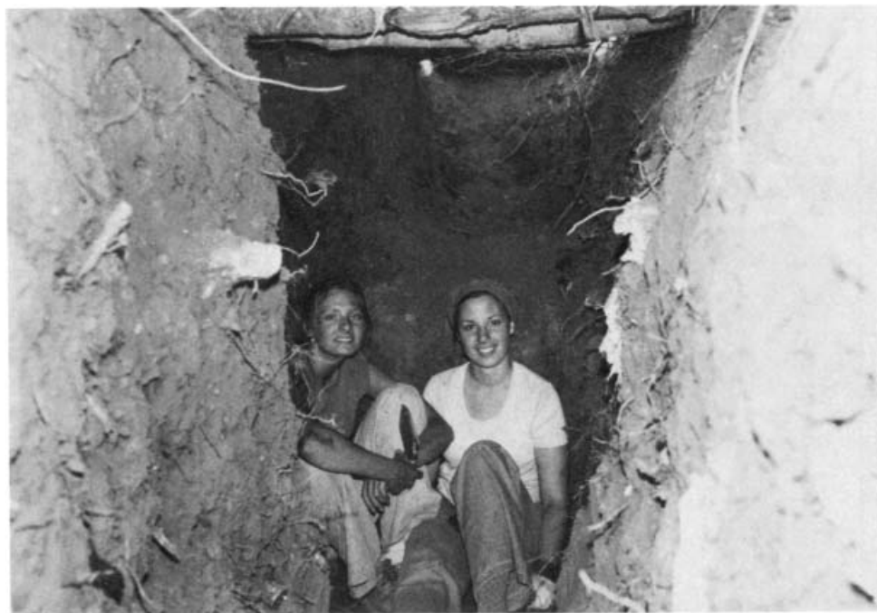
Fig. 5.2. Two non-athletic college girls who completed a 4-person Pole-Covered Trench Shelter in 35 1 / 2 hours, despite tree roots.
