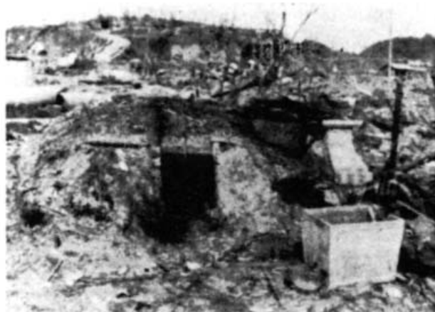
Fig. 1.5. Undamaged earth-covered family shelter in Nagasaki.
