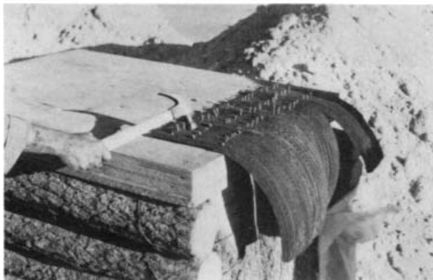
Fig. D.15. Tire-strip hinges nailed to an expedient, 4-inch-thick blast door made of plywood, designed to withstand 50-psi blast effects of very large weapons and undamaged by blast at the 53-psi range.
