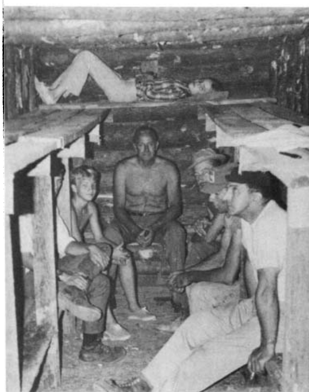
Fig. 14.2. Benches with overhead bunks in a skillfully designed Small-Pole Shelter of Russian design. Three rural families in a wooded area of Tennessee built this expedient blast shelter in 48 hours, including the time spent felling trees and making furnishings.
