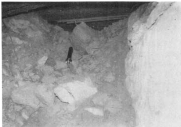
Fig. D.3. Effective earth arching in the earth covering of this 4-ft-wide Pole-Covered Trench Shelter prevented a single pole from being broken by blast forces that exerted a downward force of 53 psi (over 3½ tons per square foot) on the overlying earth.
