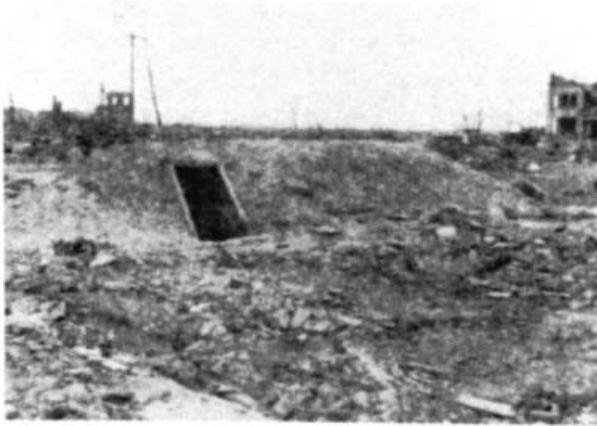
Fig. D.1. A small, earth-covered backyard shelter with a crude wooden frame—undamaged, although only 300 yards from ground zero at Hiroshima.
